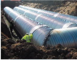
INSTALLATION OF MULTI-LEG TANK
